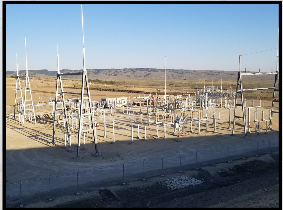
Almost done! June 27, 2018
