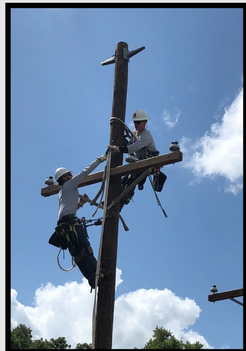
Riley and Lazy Q classmate performing "Cross Arm Change Out"
