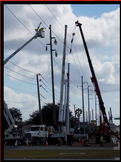
Working on a pole change along Hwy 27 in Leesburg, FL
